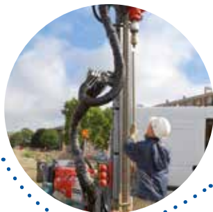
1 DRILLING AND FOUNDATION EQUIPMENT
